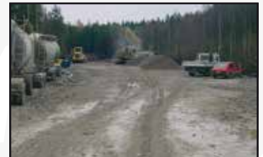
The swamp one week after stabilisation
